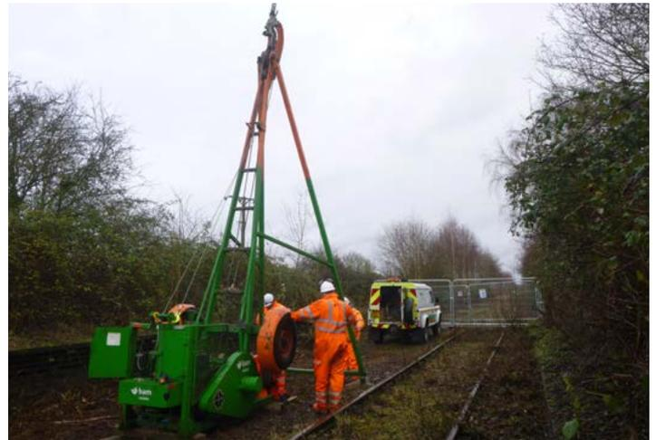
^ This cable percussive rig is being used to drill boreholes for geotechnical and water table surveys. Boreholes are typically 10 to 30 metres deep.
