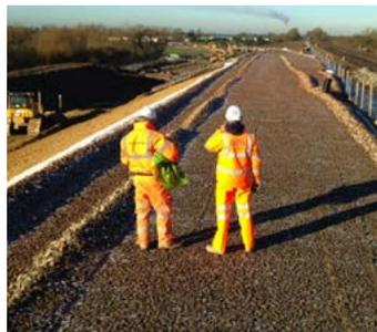
^ Bicester chord bottom ballast and track installed
