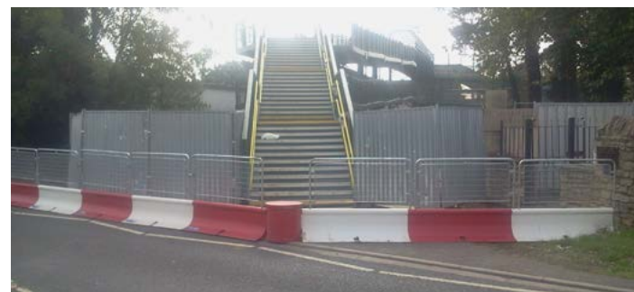
^ Scaffolding is removed from Tubbs Lane footbridge and permanent hand rails are being installed on this busy crossing for pedestrians and cyclists.
